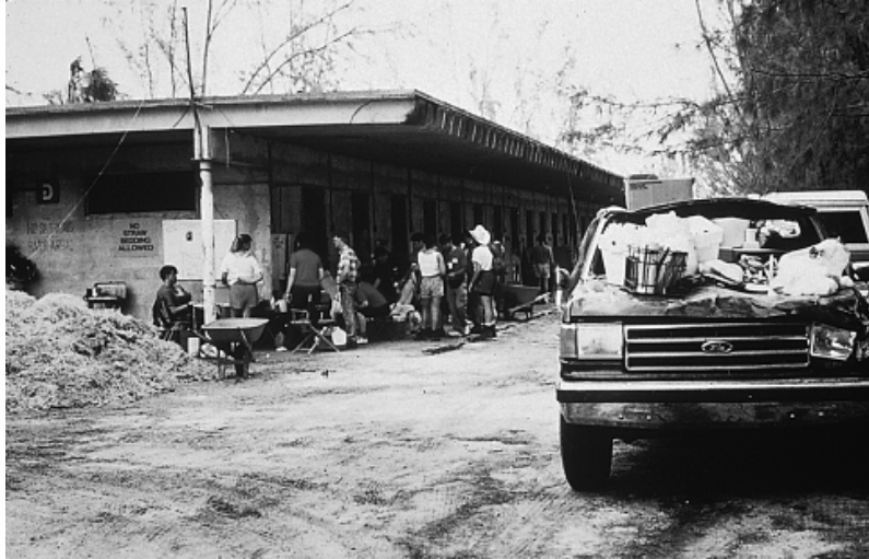
A veterinarian's truck was severely damaged when a slab of concrete fell on it. The truck had been parked overnight in the garage.
