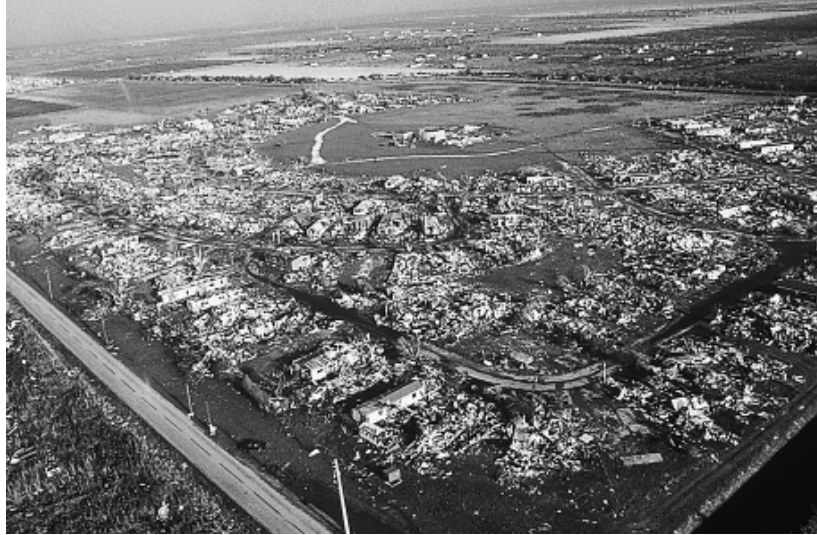
Damage to a subdivision in South Florida after Hurricane Andrew in 1992. (Photo by Rocky Bigbie.)
